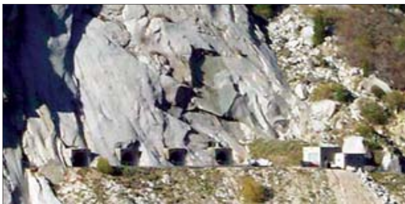
The entrances to the LDS Church's vaults, literally carved into the side of Granite Mountain in Utah. It is here that they store the millions of rolls of microfilm that are being digitized and indexed for online access.
