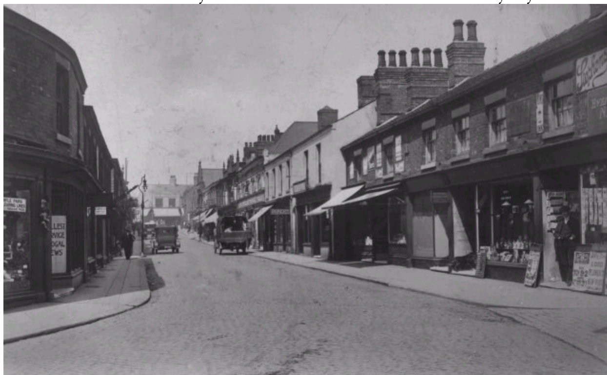
(High Street, Crewe -- Continue along Mill Street (toward the town centre) and we come to High Street. In the distance we can see the junction with Edleston Road.) 2
